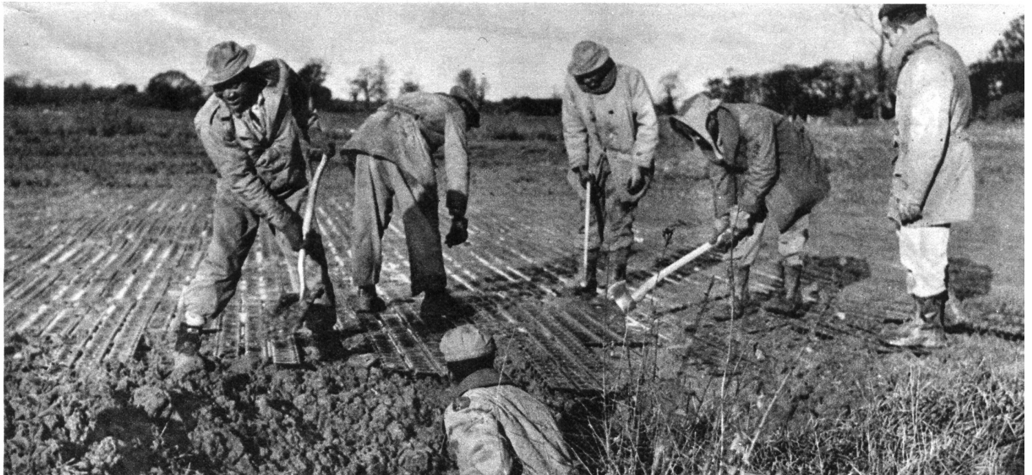
10 While repair job is under way, members of engineering unit level off ground, fill ditches and fix metal landing strips so that Fortress can take off when repairs are completed. Soft ground which enabled an easy landing would have endangered take-off.
