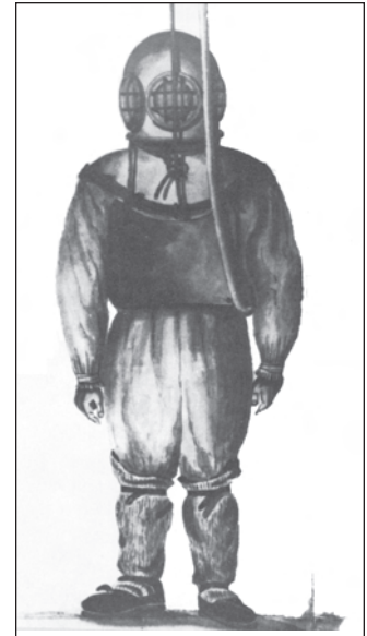
Figure 1-5. Siebe's First Enclosed Diving Dress and Helmet.
