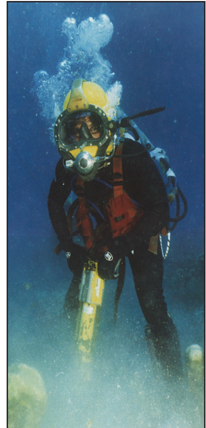
Figure 6-4. Underwater Construction Diving.
