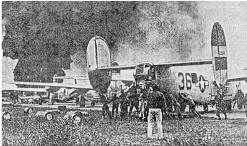
The 461st Bomb Group was unloading ferried gasoline in southern France when a spark ignited a load of fuel and flames consumed this aircraft. Crewmen strain to swing another Liberator around and out of danger.
